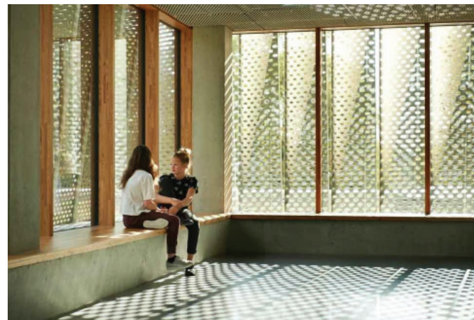
FACADE IDEAS - LASER CUT METAL SHEET SCREEN
