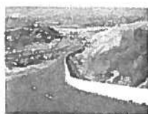
5000ft of Sterndahl K rail along the 14 freeway
