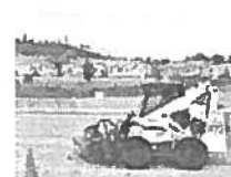
Bobcat removes rpm stripes
