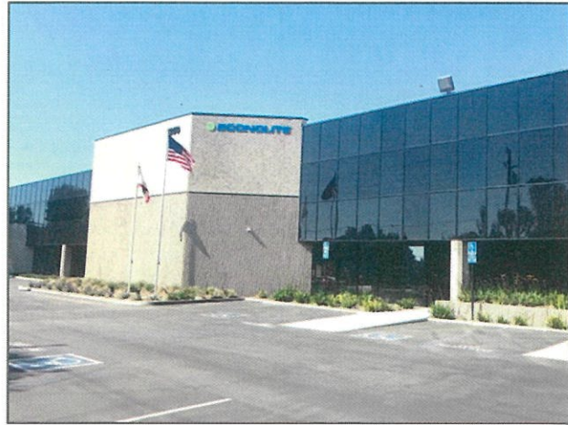
Figure 4: Local Support - Econolite's Headquarters in Anaheim, CA
