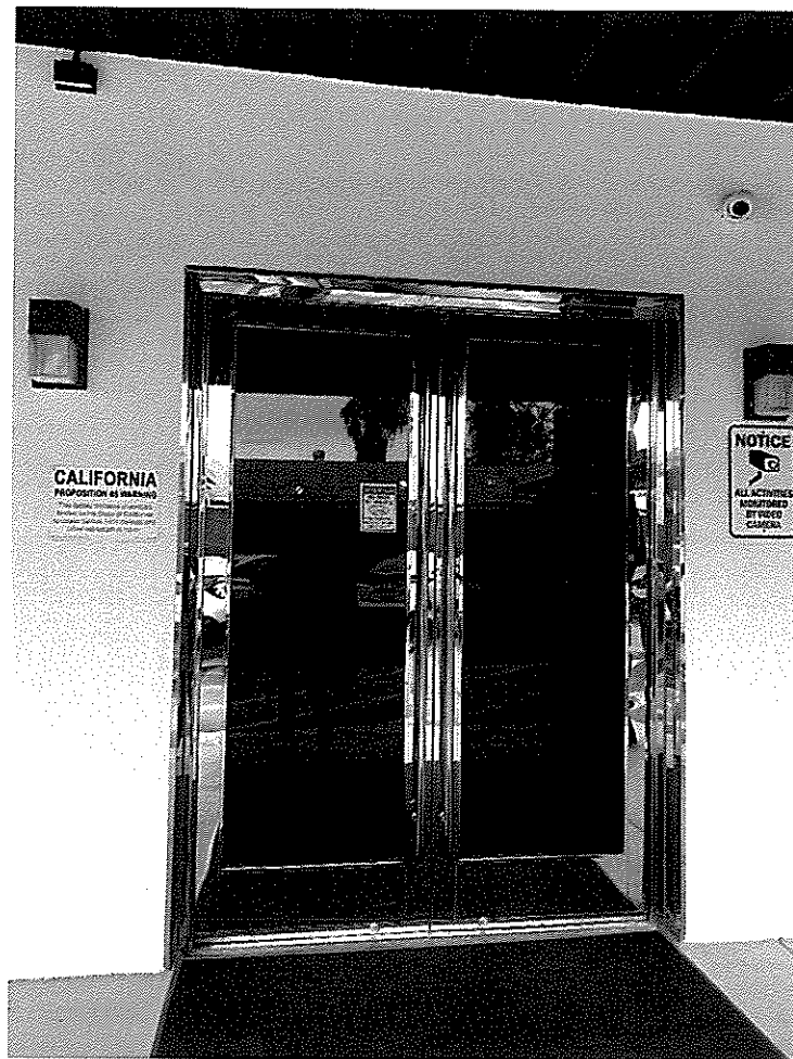
QR Code certificate not displayed clearly visible from the outside of the licensed premises. (Exhibit 1)
