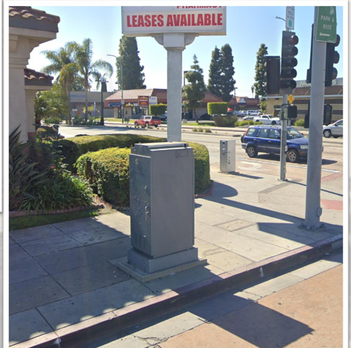
Example of unpainted signal box
