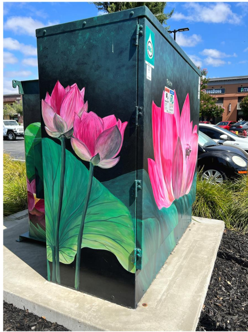
Example of box painted in place
