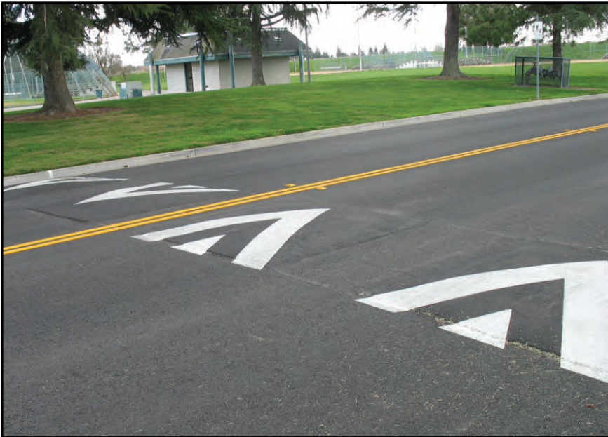
Example of potential Speed Cushion treatment
