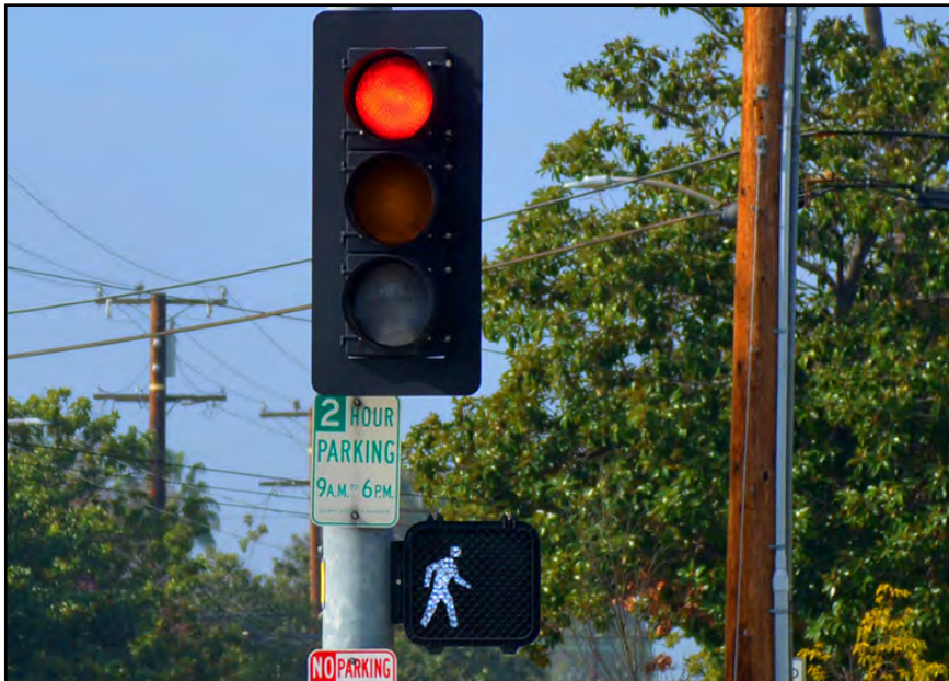
Example of LPI indicating pedestrians to cross before traffic is allowed to move
